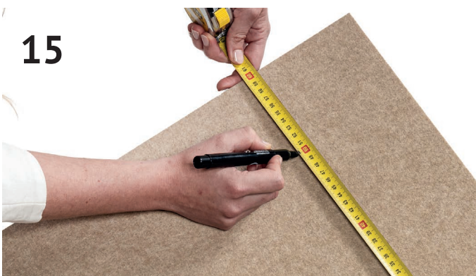
15 Mark a dot 10 centimeter from the upper edge on the right side
