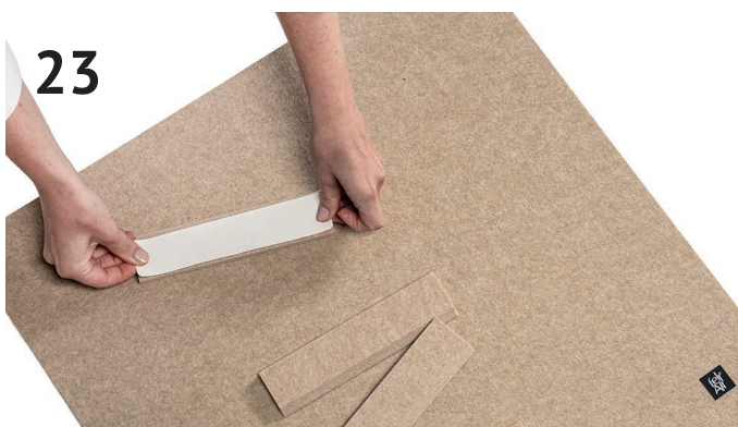
23 Position the double sided tape to the back of the felt spacer
