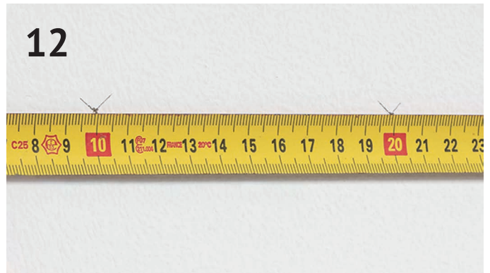
12 Double check if the distance between the two drilling points is 10 centimeter
