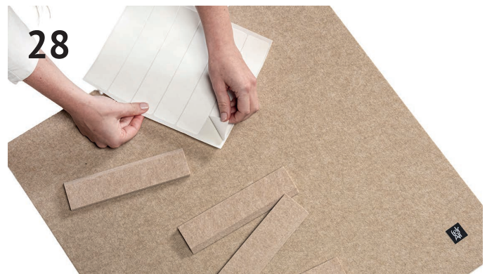
28 Option 2: Use double sided tape (enclosed sheets) Check the data sheet first
