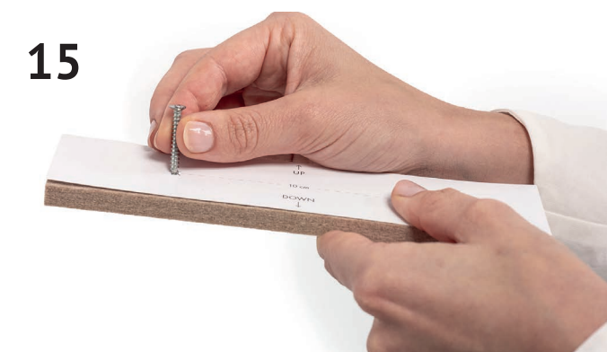
15 Mark the 2 drilling points (X) by pressing a screw firmly through the paper
